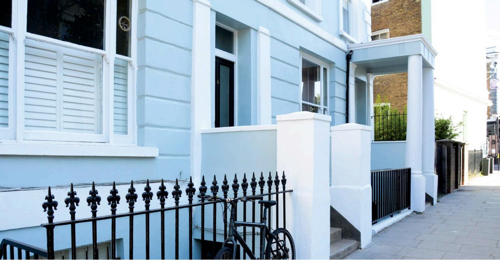
The scope of Exterior Works included roof works (including leadworks to dormer roofs and loft insulation); repair and painting of timber windows and replacement of some windows with double glazed uPVC/timber windows; brick work including render repairs, cleaning and painting; and guttering and pipework repairs including painting all guttering.
