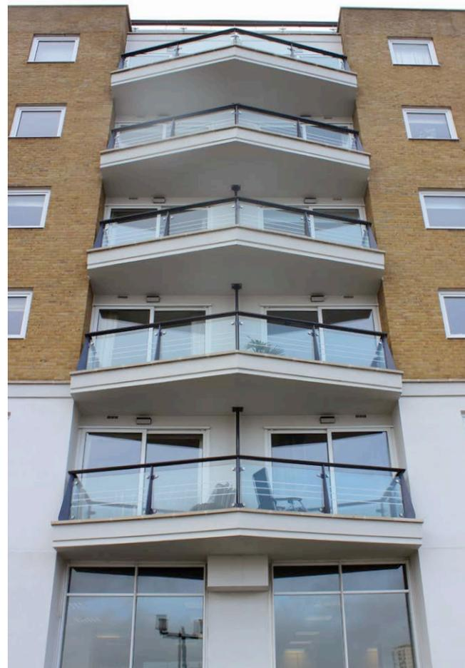
Brick works included hacking off and repairing damp and stained render and bricks as well as cleaning external brick work and coping stones using the DOFF cleaning method. We also painted external brickwork.
